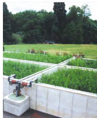
Station de Ligny-le-Ribault, Loiret
